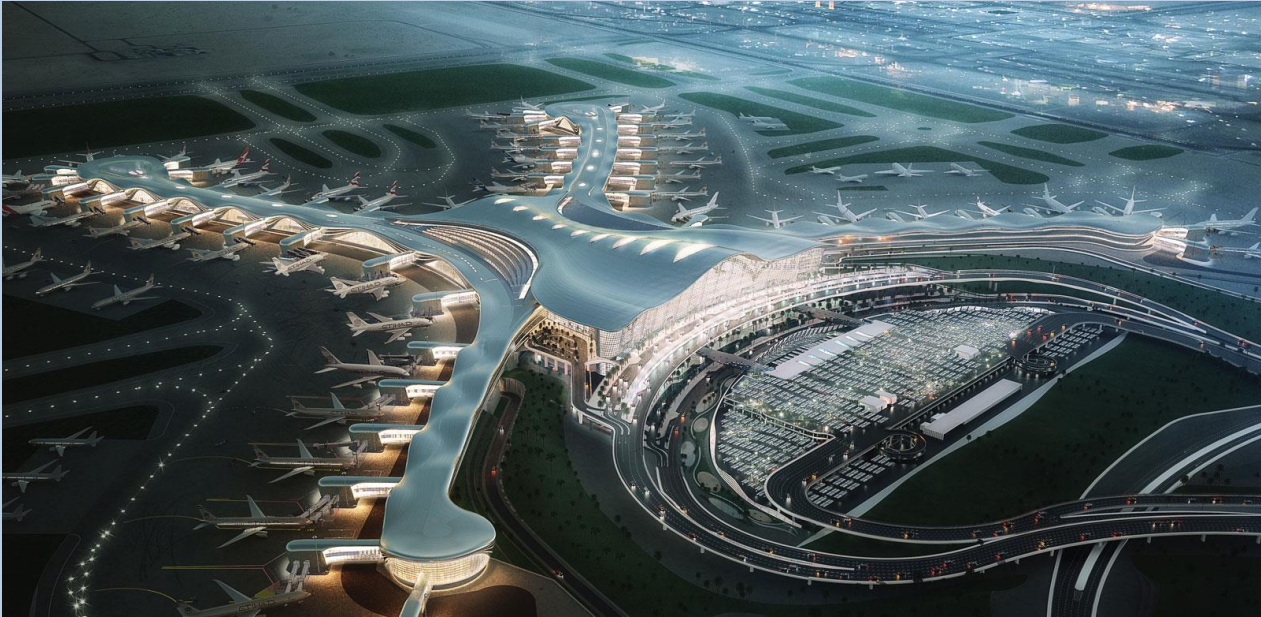
Exhibit 10: Abu Dhabi’s New Midfield Terminal (Exterior Above, Interior Below)
